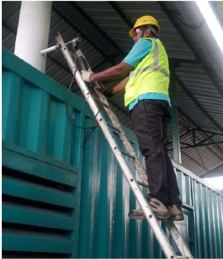
Flue Gas Monitoring GG # A SL. No.: GZC-00228
