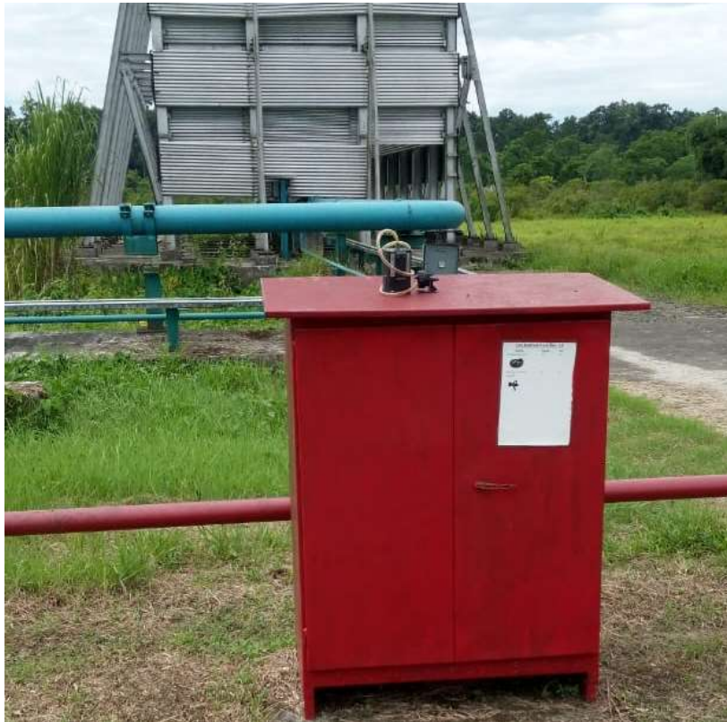
Ambient Air Quality Monitoring HMGPP, AREA 60 (Near Fire Extinguisher Cabinet)
