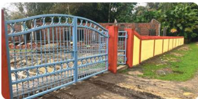
Boundary wall construction at Lama Goan Middle School, Assam
