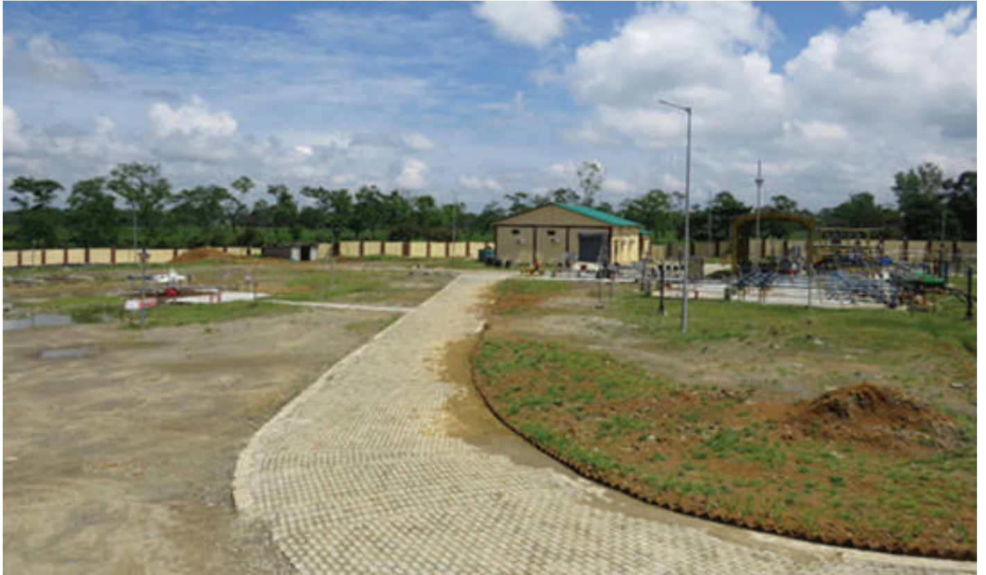
Drill site restored at GGS of Assam
