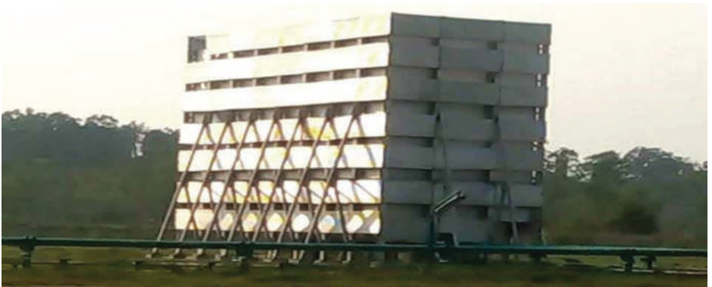
Flare Enclosure at Modular Gas Processing Plant in Assam
