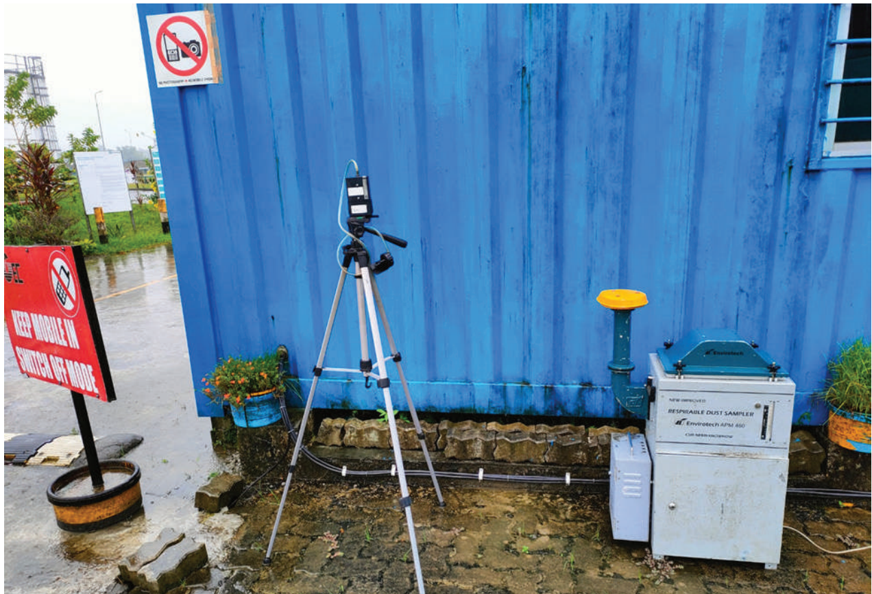
Air quality monitoring by PCB accredited agency at MGPP
