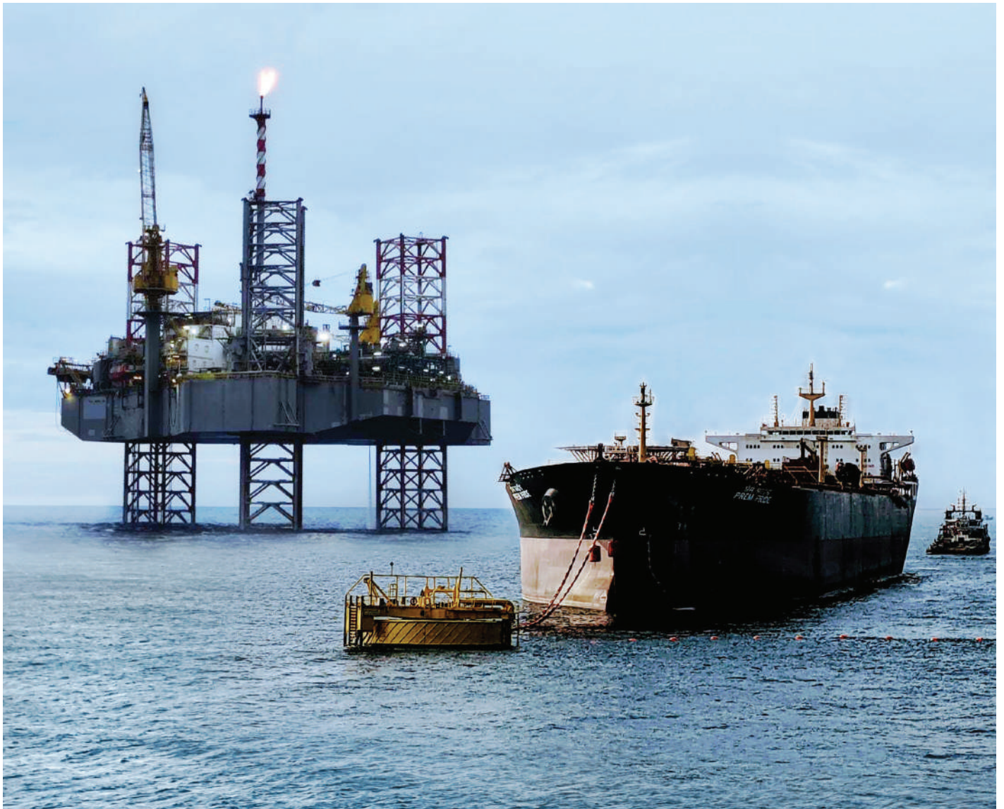
B-80: KGB-Offshore Installation with FSO and Calm Buoy
