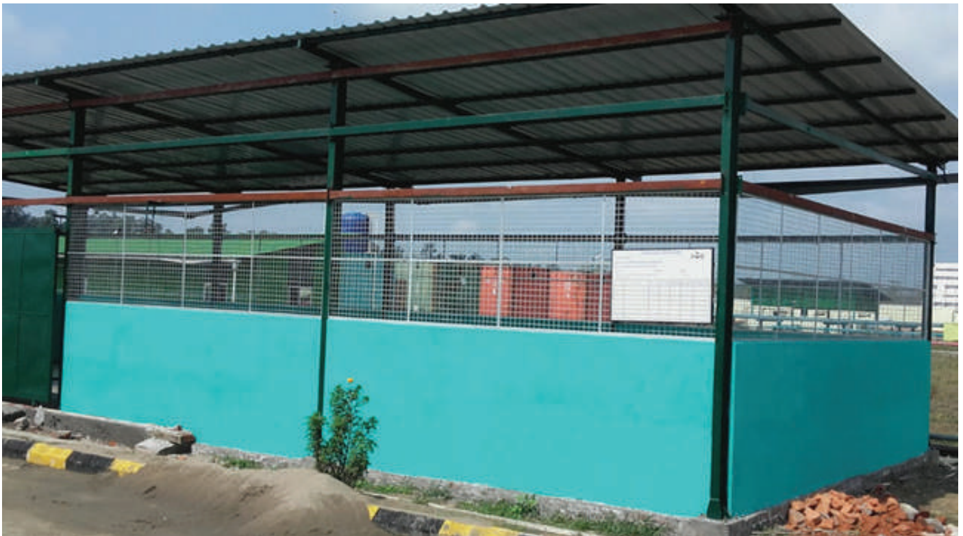
Hazardous waste storage yard at MGPP with ventilation
