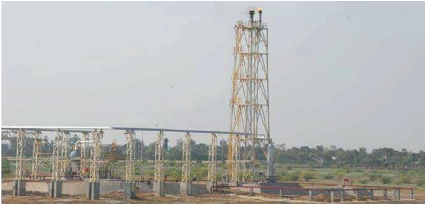
Flare Tower at PY-1
