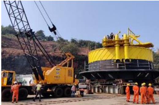
Single Point Mooring (SPM) System
