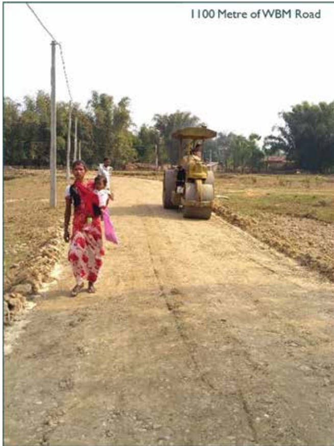
Figure: Construction of New WBM Road in Augbandha Village
