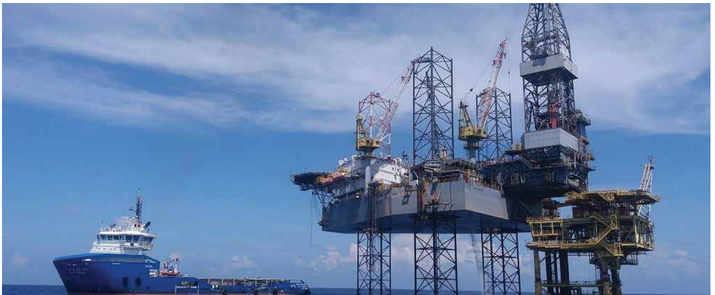
Figure: PY-1 Offshore Facility & Rig during Drilling Operation
