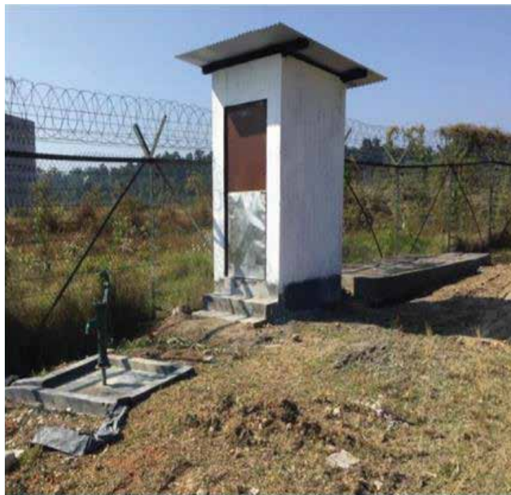
Figure: Construction of New Public Toilet in Augbandha Village
