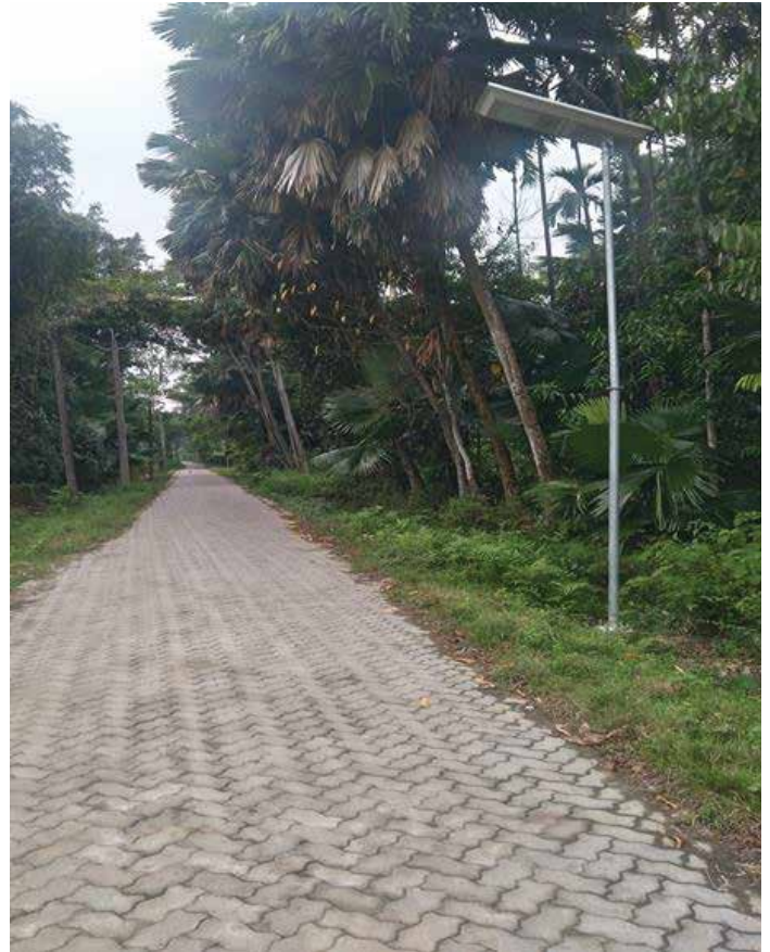
Figure: Construction of New Cement Block Road in Augbandha Village
