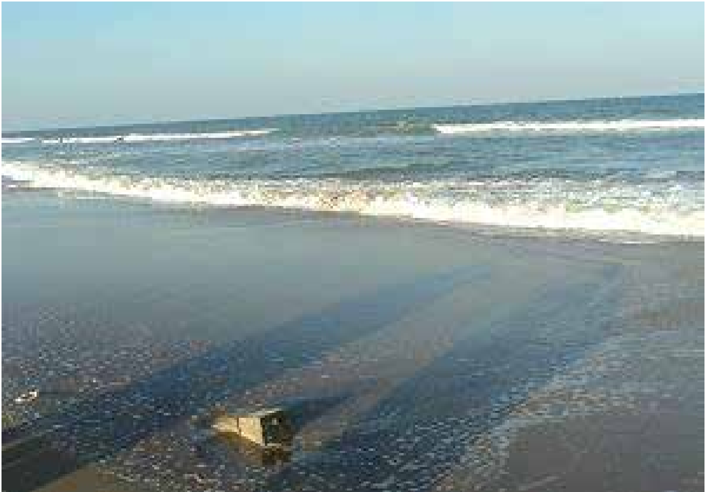
Figure: Marine Outfall Point at PY-1
