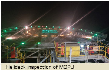
Helideck inspection of MOPU
