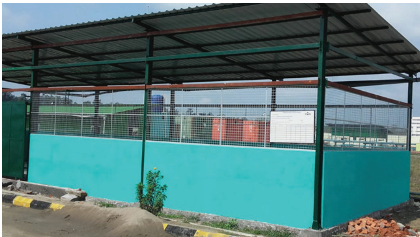
Hazardous waste storage yard at MGPP with ventilation
